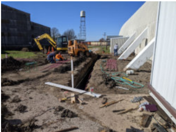
Digging the footings (K. Drewelow photo)
